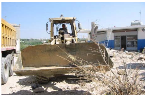
Work underway in 98 municipalities in Southern Lebanon to clear the rubble
